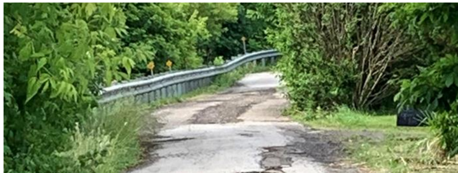
Figure 3-1 Site Photo of Tallman Drive - Example of Guide Rail Deformation and the Deteriorating Roadway
